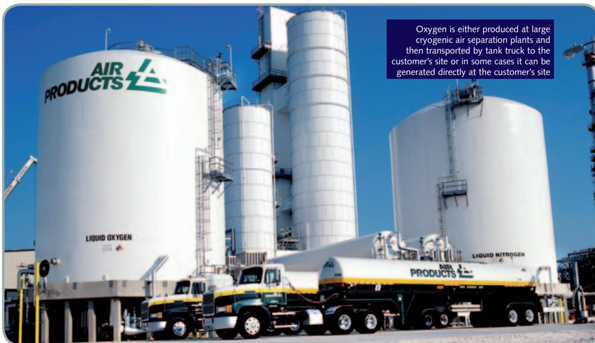
Oxygen is either produced at large cryogenic air separation plants and then transported by tank truck to the customer's site or in some cases it can be generated directly at the customer's site
