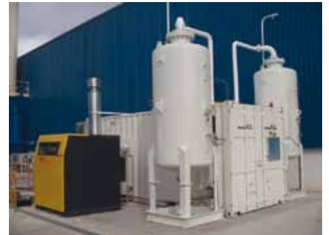
Halia® Propeller Aeration System
